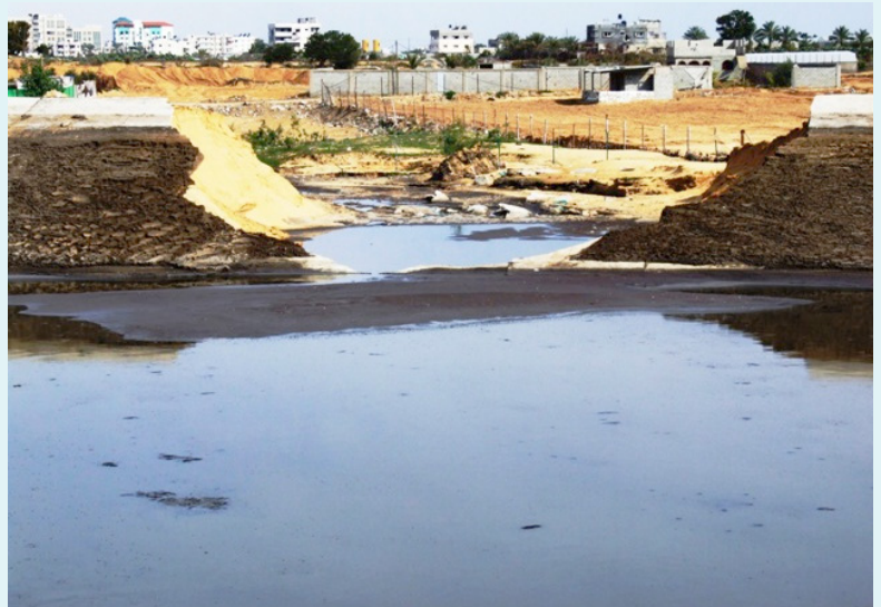
Fig.10 Bombed Water Purification Plant, Gaza City. Photo EWASH.
