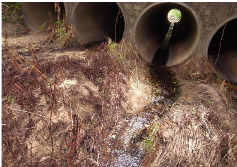
Fig.3 Storm-water drains under road crossing. Moolabin Creek, Qld, March 2014. Photo by author.
